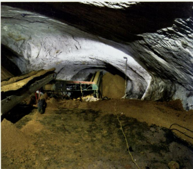
London Road mine in August 1987: backfilling in progress. The height and roof-span of this part of the mine can be appreciated (the conveyor belt is two to three feet wide. Photo Nick Catford.
